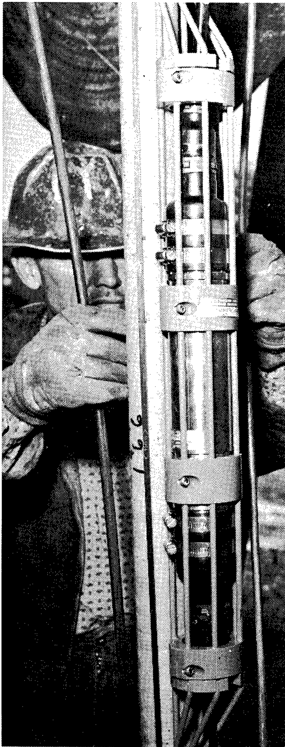
Fig. 3. Instrument being lowered in hole GB-1. Grout was pumped through the fiberglass pipe to which the instrument is attached to provide coupling with the formation.
