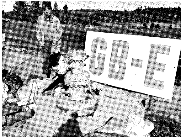
Fig. 1. GB-E well-head installation immediately after reentry, about 3 hr after shot time. The area is being checked for the presence of gaseous radioactivity; none was found.
