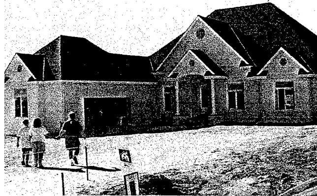
Figure 1-1. New ICF Home in Wisconsin [icfweb.com, 2000]
