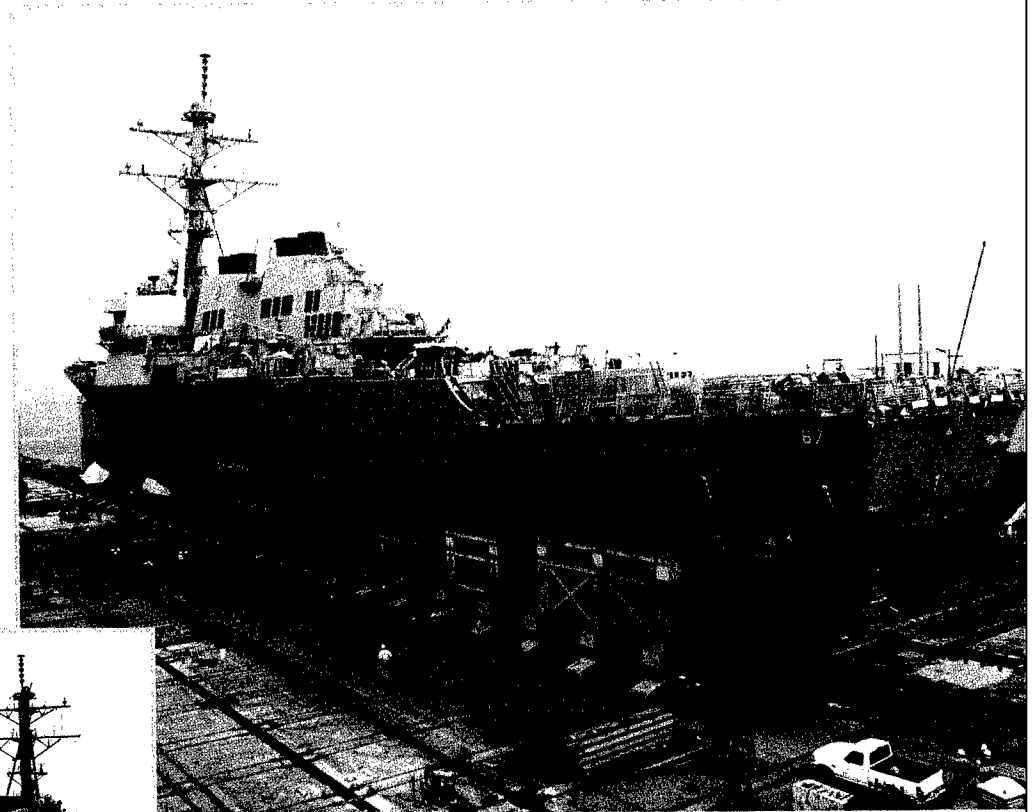
▲ USS Cole moved on land from Litton Ingalls Shipbuilding's floating drydock Jan. 14. The 8,600-ton destroyer moved at a pace of 27 inches per minute, covering the 100-yard move from the water to a construction area inside the yard in less than three hours. The ship will remain on land for the remainder of its restoration. (Litton Ingalls Shipbuilding)
