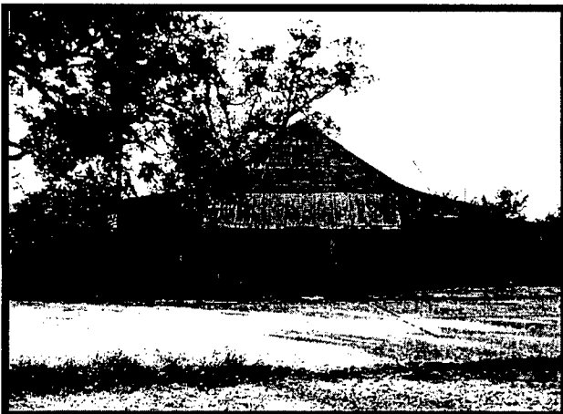
Figure 122. An overview of the front (western) elevation of Standing Structure 55-1013. Note the front-gable, the side wings, the window in the gable wall, the horizontally oriented plank cladding, the front porch, and the awning covering the front porch.
