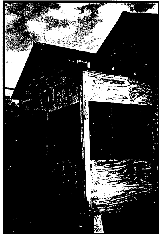
Figure 92. A detail of the front porch at Standing Structure 55-1112. Note the plywood cladding.
