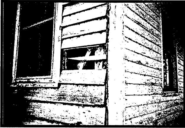
Figure 77. A detail of the northern elevation of Standing Structure 55-1113 depicting the wood frame, braced frame construction. The braced frame can be seen in the section where the wooden planks have been removed. Also note that the horizontally oriented wooden planks are lapped.
