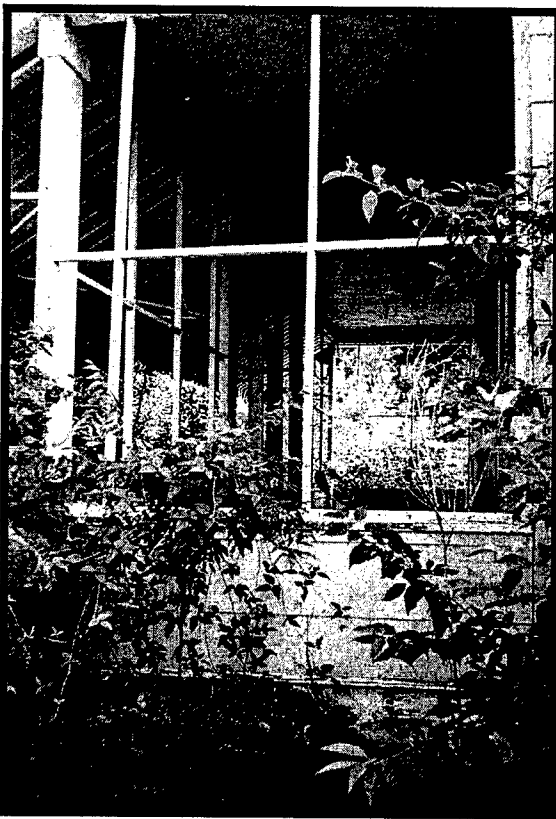
Figure 114. A detail of the front porch at Standing Structure 55-1012 facing north. Note the porch columns and the attached wood frame designed to support screening.
