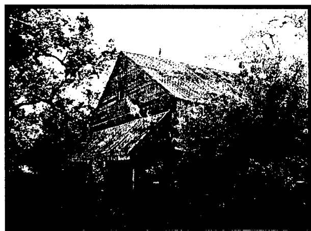
Figure 123. A second view of the front (western) elevation of Standing Structure 55-1013. Note the front gable, the corrugated metal roof, the vertically oriented plank cladding, the window in the gable wall, the front porch, and the awning covering the front porch.
