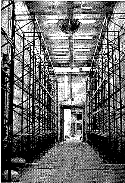
Photo 4. One of 20 compartments with space for 192 pallets
