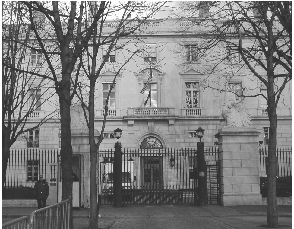
Figure 6: Vehicle Entrance to the Embassy
