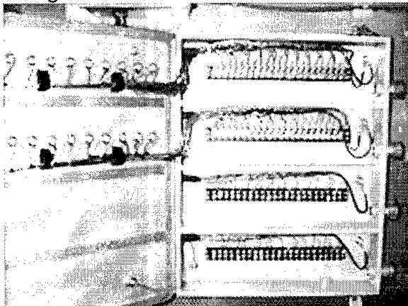
Figure 2. Electrical Penetration Port
