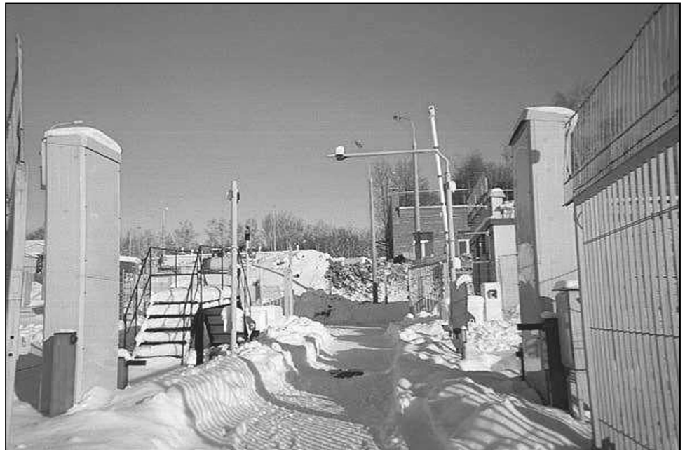
Figure 3: Security Assessment and Training Center in Sergiev Posad, Russia
