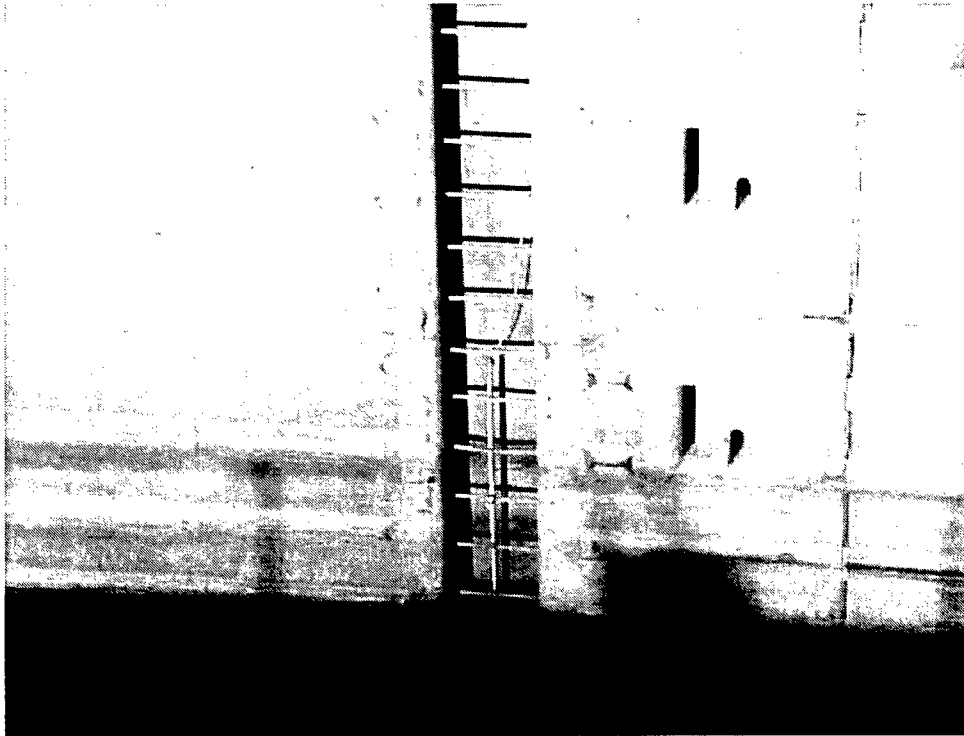
Figure 5. Lower pool pressure transducer location in the ladder well recess on the land wall
