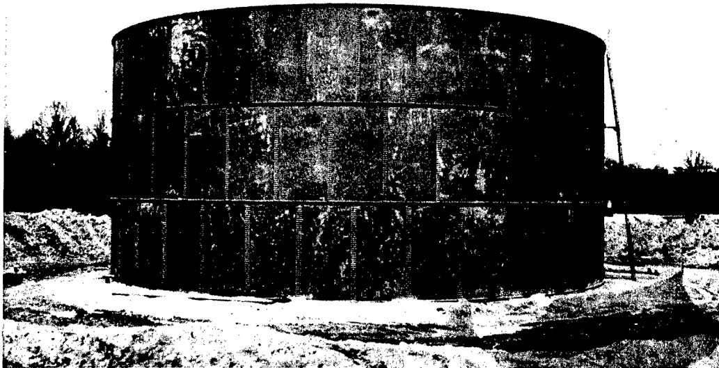
Fixed 10,000 bbl. bolted steel tank for fulk storage.
