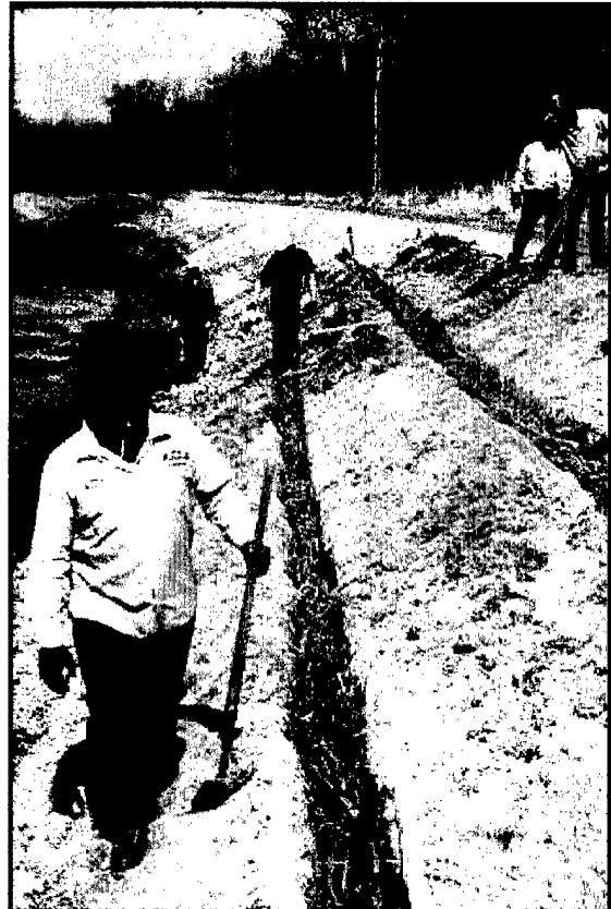
Figure 3. Installing a live fascine structure
