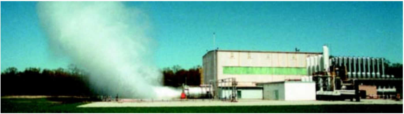
Aeropropulsion Test Unit creates hypersonic test conditions.
