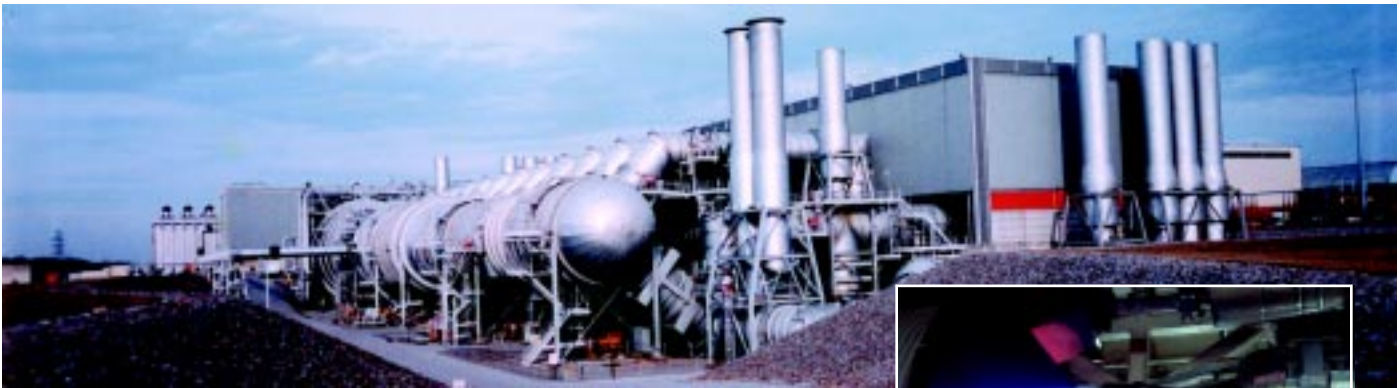
Aeropropulsion Systems Test Facility tests large turbofan commercial and military engines under simulated flight conditions.
