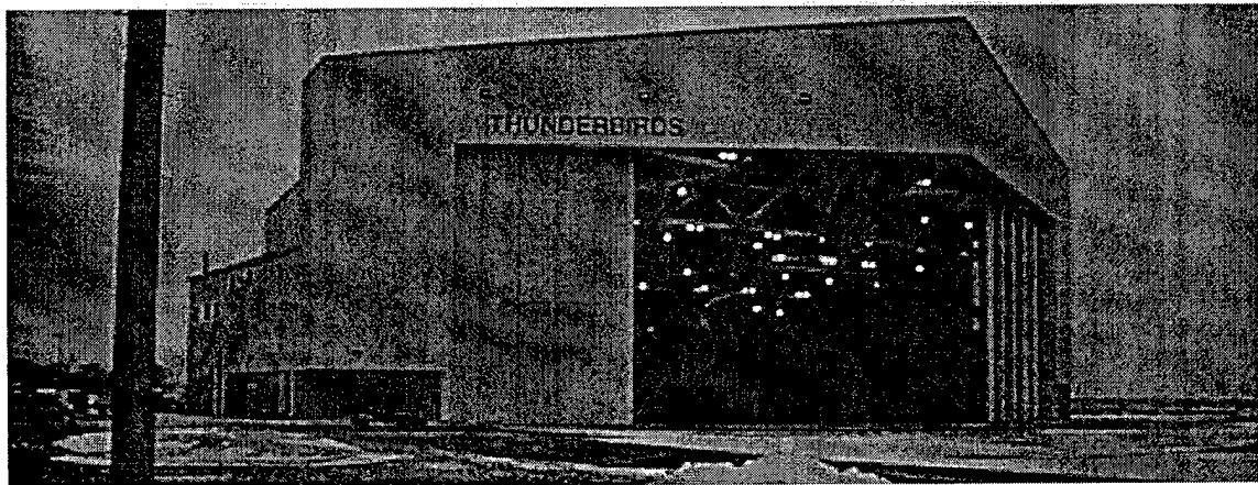
Figure 3. Front (South) Face of Building 198, Mountain Home AFB.
