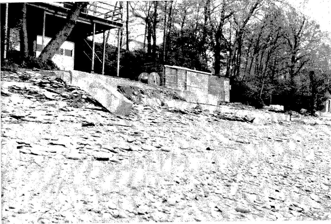
Figure 22. Cottage with protective concrete blocks east of the location shown in previous figures, 17 May 1991. Note the block that has been moved by storm waves. The three properties in the foreground are vulnerable to storm waves because they were built on the beach rather than up on the bluff like the house in the background. Photograph from Buffalo District archives
