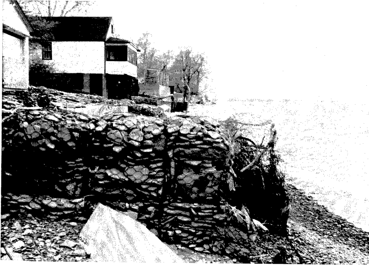
Figure 21. Gabion wall east of property shown in previous photographs, 17 May 1991. Leaning tree where concrete block walls are found is in distance. Photograph from Buffalo District archives
