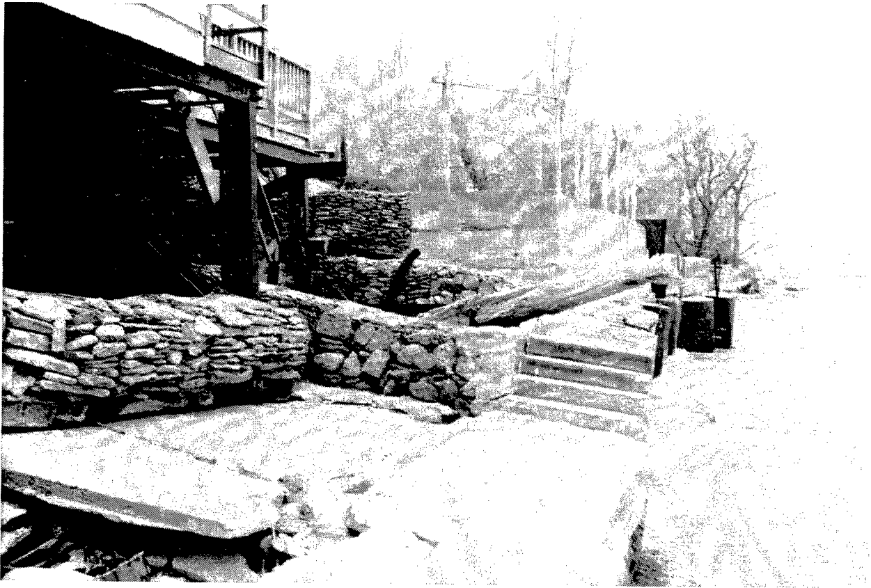
Figure 19. House protected with gabions, concrete, and concrete-filled tanks, May 1991. These structures are about 500 m east of marina's east wall (visible in right side of photograph). Notice tree trunk resting on wall next to steps, evidence of power of storm waves. When this photograph was taken, there was no beach at base of concrete slabs. Photograph from Buffalo District archives
