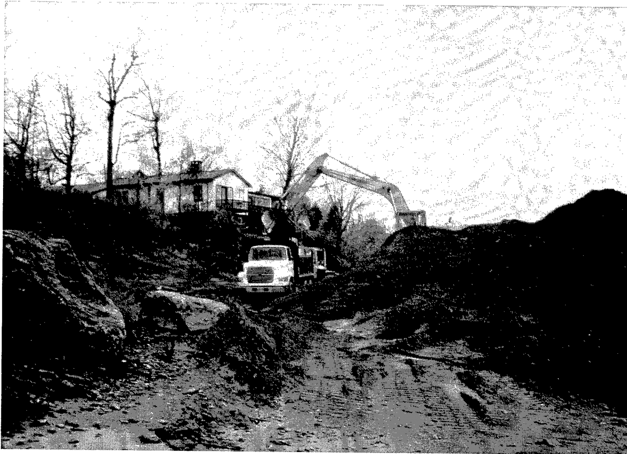
Figure 25. West fillet sediment being loaded into dump trucks, 17 November 1998
