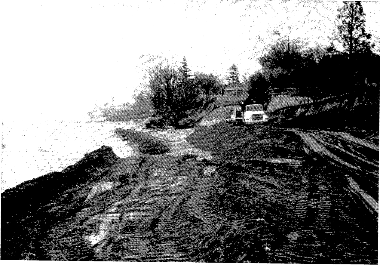
Figure 27. Temporary road along base of bluffs east of marina, 17 November 1998. Sediment is spread across beach and into water by a bulldozer
