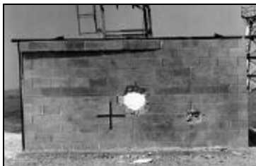
Filled Block Wall
