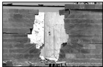
Cinder Block Wall
