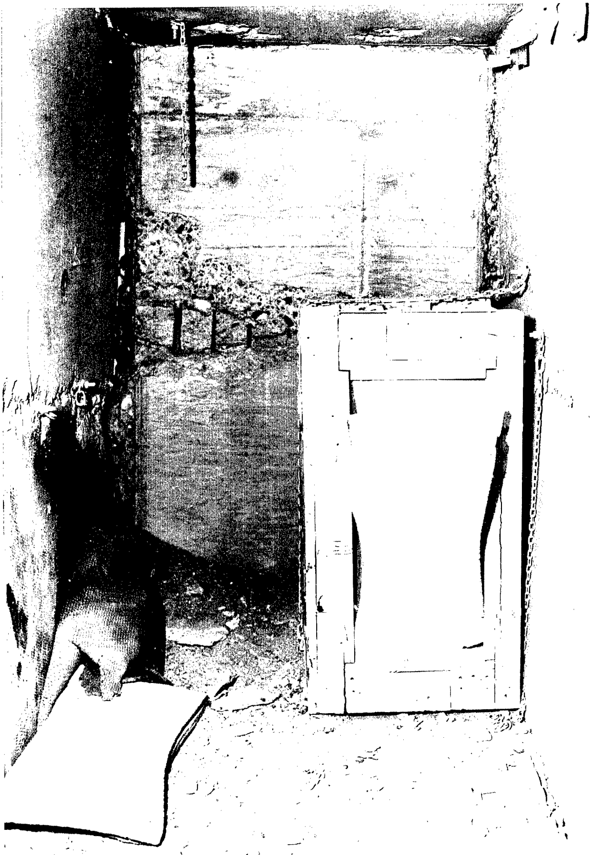
Fig. 4.9—Trap 1A, postshot, half-size trap in basement exit shelter (34.1 d-2) with open door, 1470 ft from Ground Zero.
