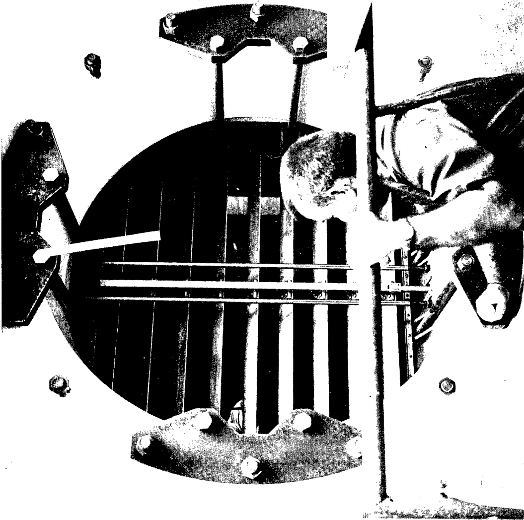
Figure 2.5. --Installed louver blast valve as viewed from air shaft, PRAIRIE FLAT Event.
