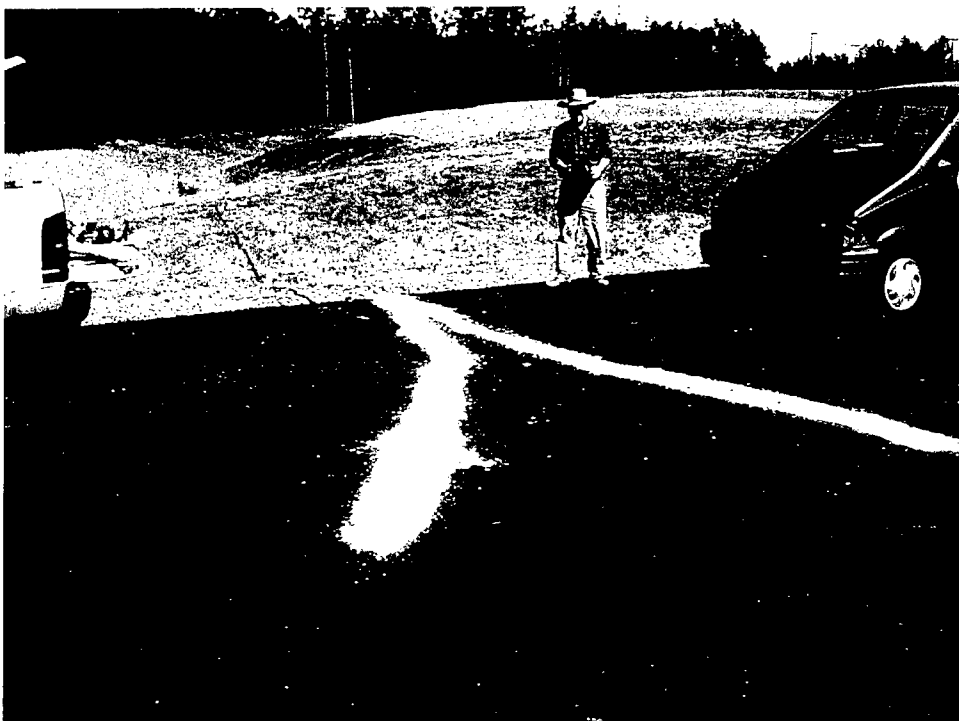
Photo 22. Trench on top of upper binder course, covered with fine aggregate
