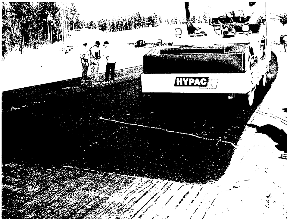
Photo 16. Compacting ropes into asphalt concrete to form temperature probe trenches
