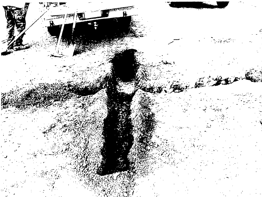
Photo 11. Trench for installing 2 Sentry 200 moisture probes, along with a CS615 moisture probe
