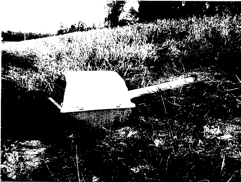
Photo 28. Doghouse enclosure for a tipping bucket
