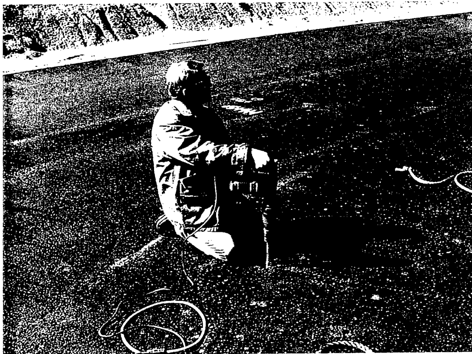
Photo 18. Drilling down to bottom of upper binder course
