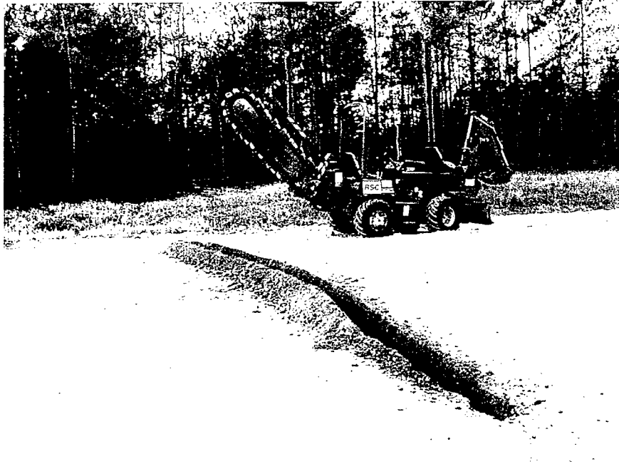
Photo 10. Trench for installing a CS615 moisture probe
