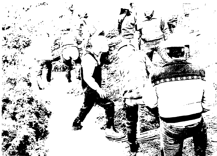
Figure 5. Installation of vertical willow bundles landward of juniper tree revetment; the tree revetment served as toe protection between two barbs and promoted sediment deposition
