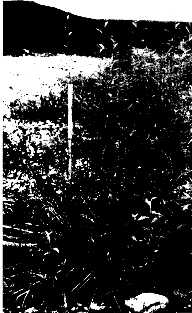
Fig. 11. Individual brush bar 6 years after construction, with feltleaf willow growing from sprouted buried branches (meter stick in photo for reference).
