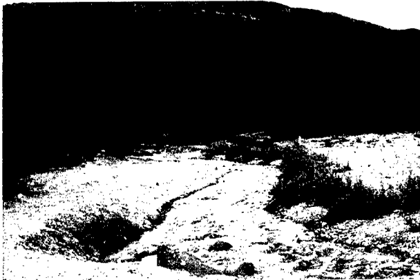
Fig. 10. Brush bars along channel reach (shown in Fig. 9) 6 years after installation. Note that vigorous willows and other plants are growing in and around brush bars.
