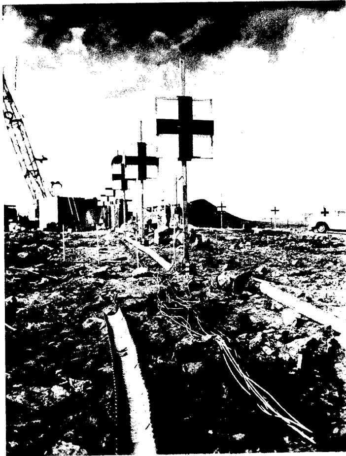
Figure 2.4 View toward SZ showing instrument cables.
