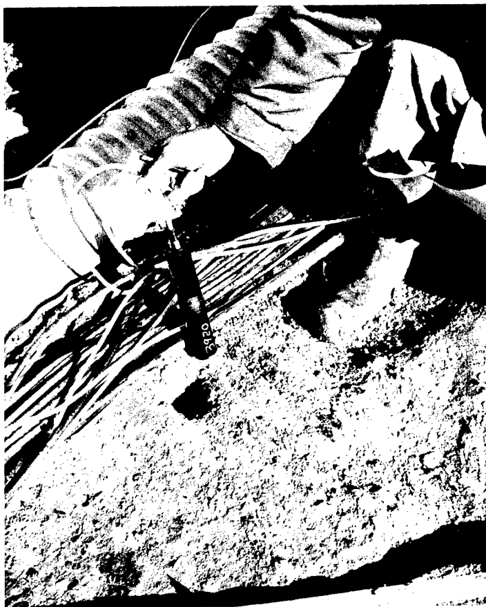
Figure 2.8 Velocity meter installation.
