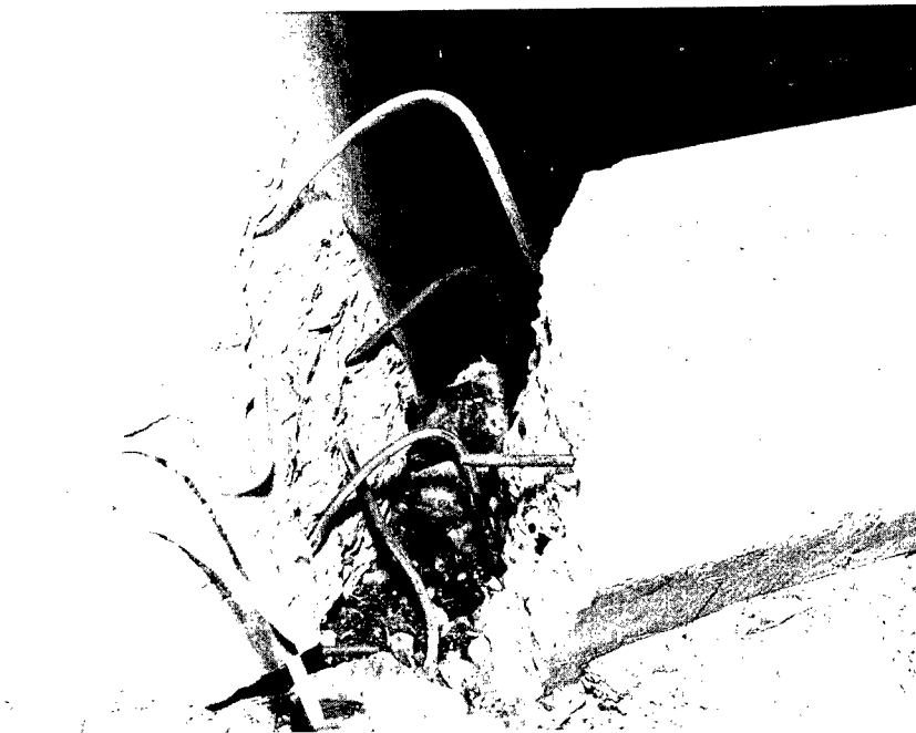
Fig. 3.19—Detail of crack at intersection of interior wall and parapet wall facing toward GZ (structure RAa).
