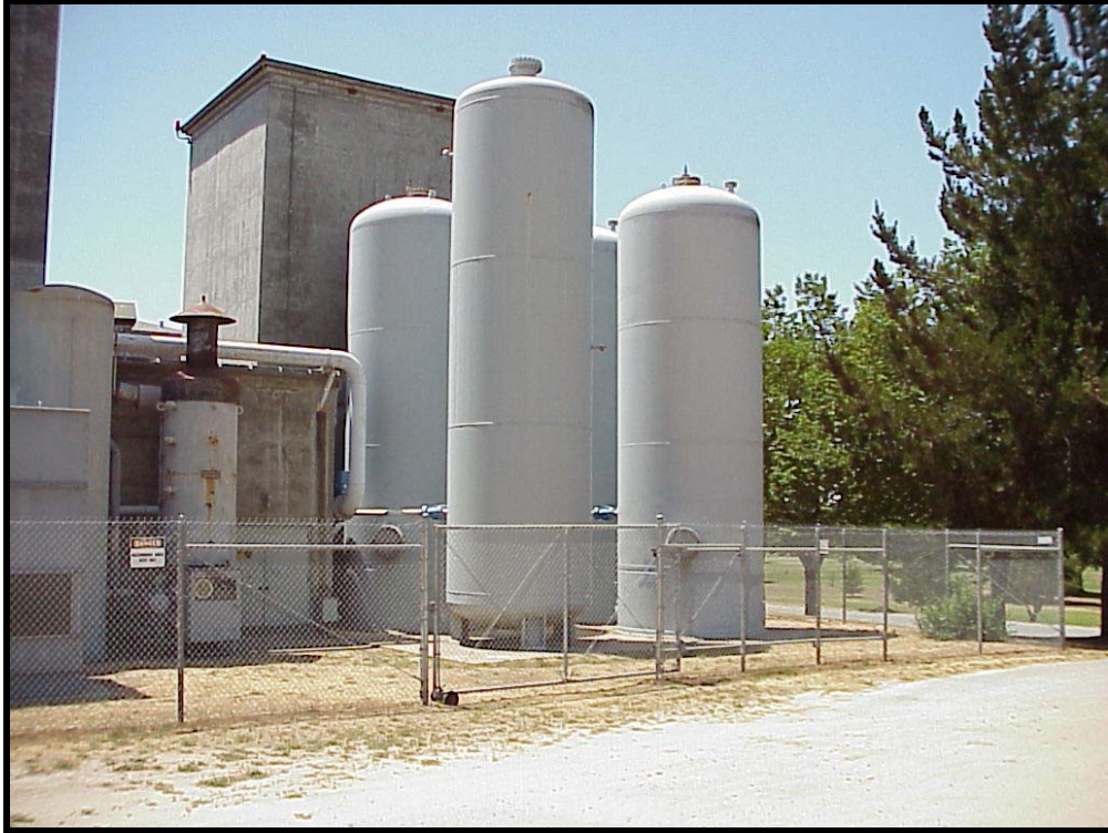
Figure 2.5. Gas dynamics laboratory tank farm.
