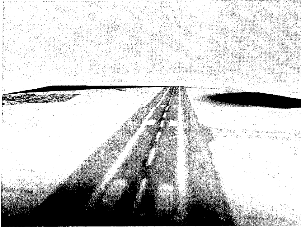
Figure 14 Eglin Damage Runway
