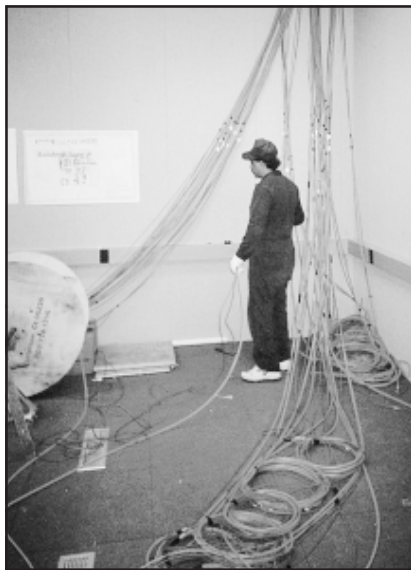
Installing fiber optic lines
