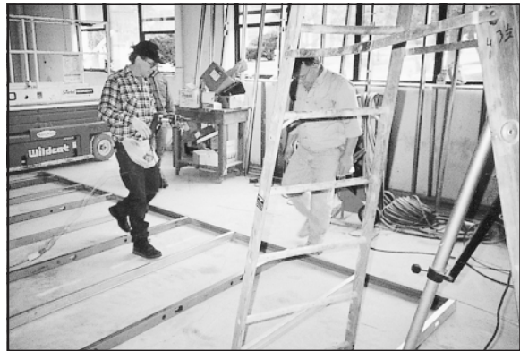
Installation of Research Facility
