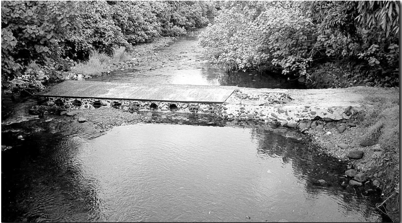
Figure 7: FEMA Assistance (Bridge Replacement) in Pohnpei, FSM
