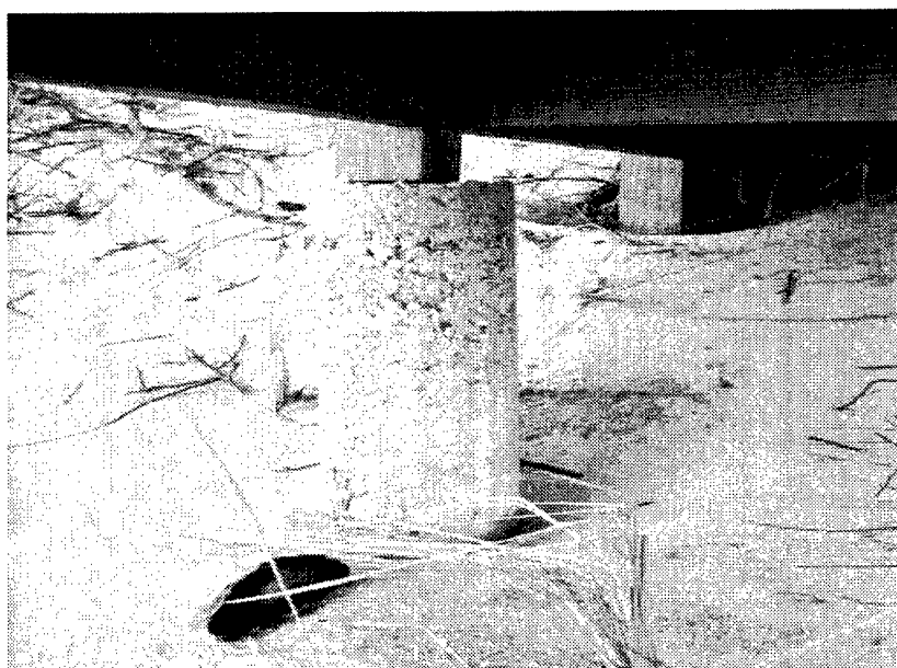
Figure 18. Wind scour around elevated dune walkway
