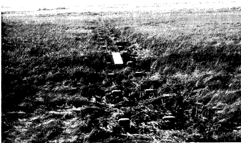
Figure 21. Stub pilings used for saltmarsh walkway
