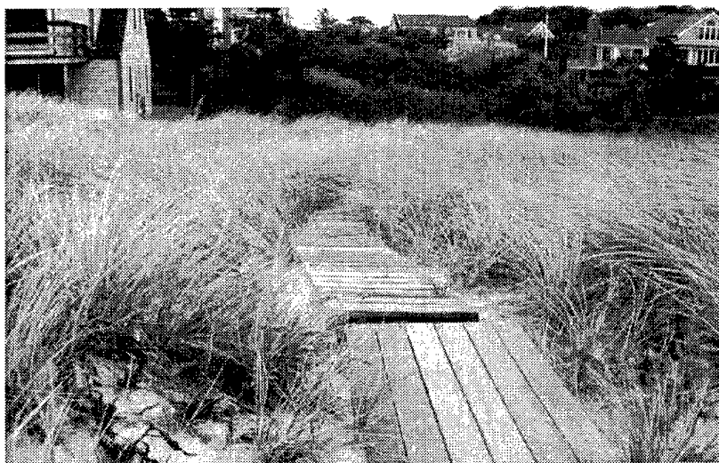
Figure 19. At-grade dune walkway
