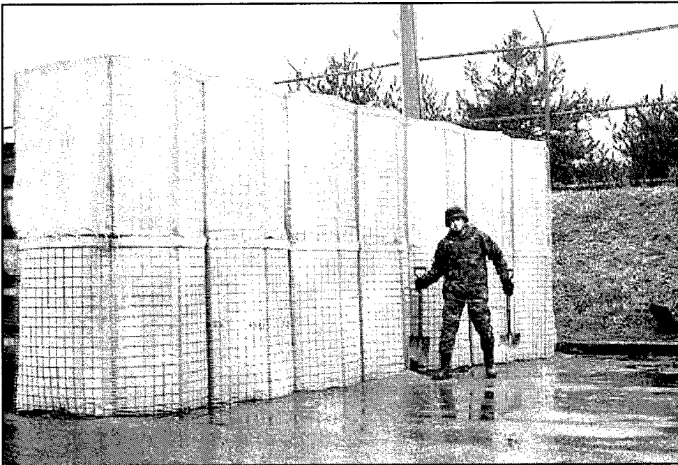
b. Completed wall
