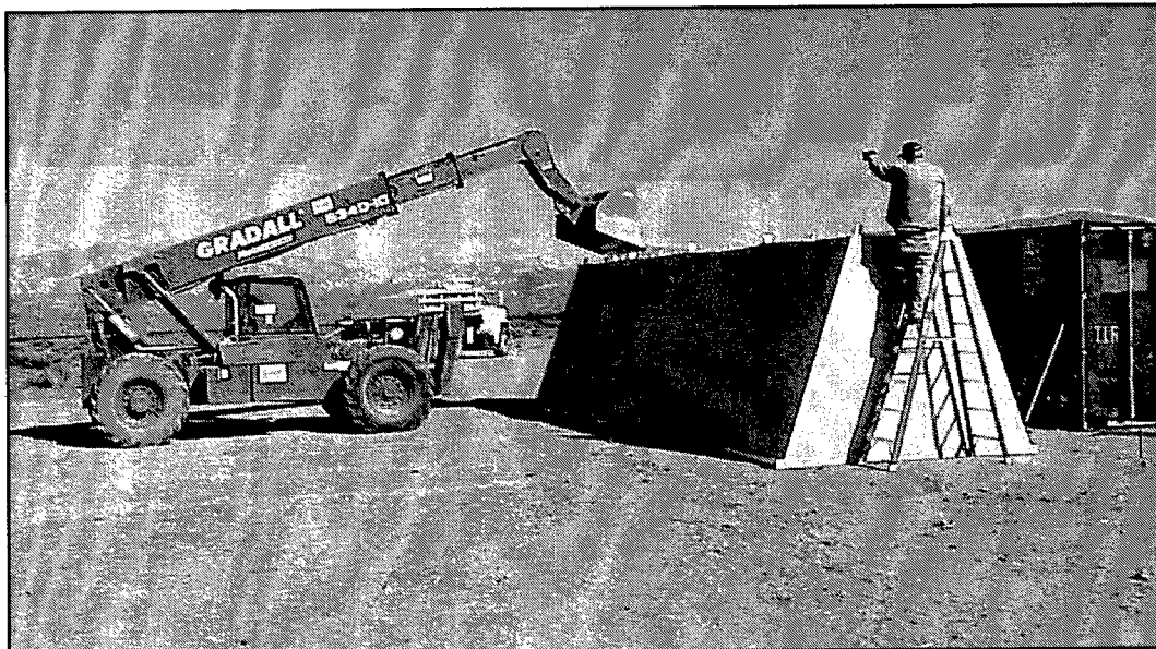
b. Dumping sand into wall enclosure
