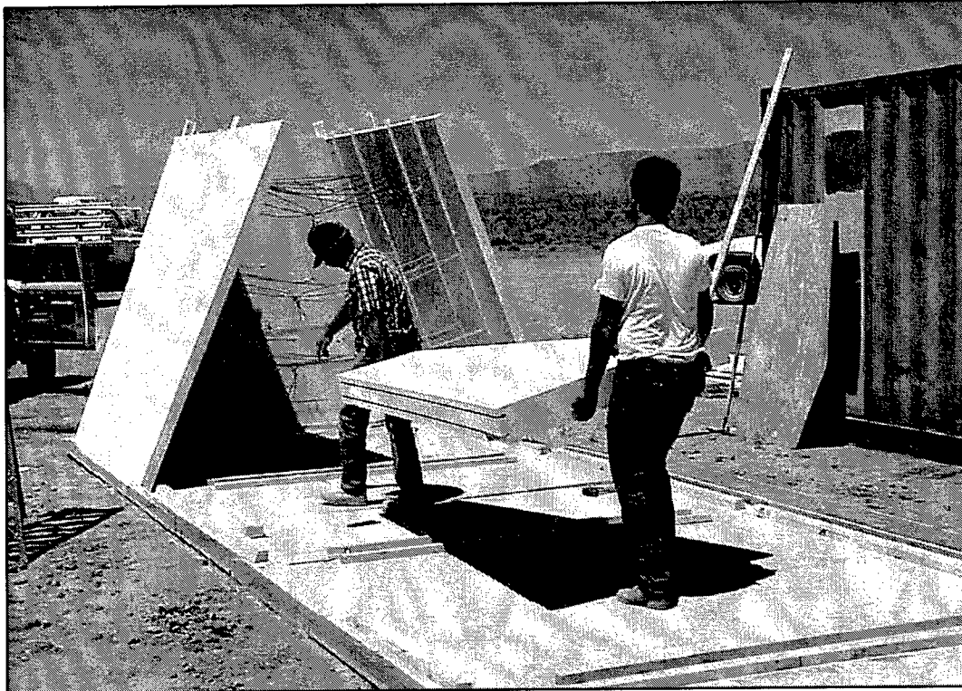
a. Erecting wall panels
