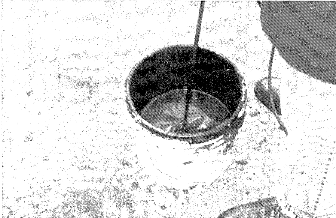
Figure 3.7 Mixing sealer components to a uniform consistency.
