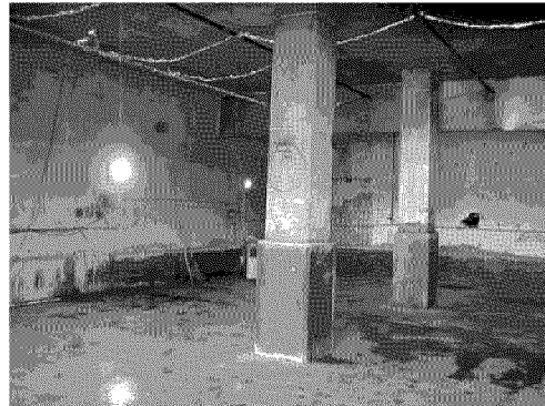
Figure 2: NATO Facility Test Room
