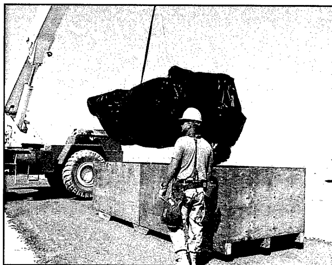
Figure 5. Bladder Getting a Lift
