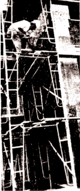
End frame not guarded. NOTE: The hole between the scaffold planks is large enough to fall through (left).
