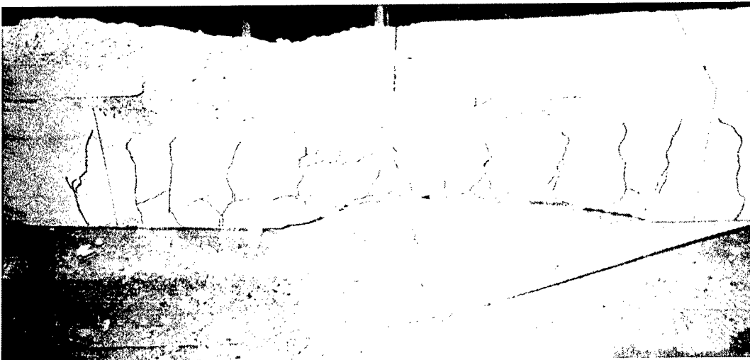
I-8-Y-AL32 crack pattern in the moment span
