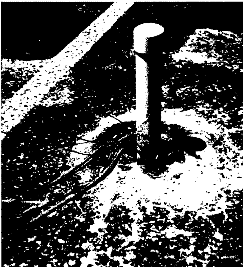
Photo 9. Oxygen sensor/VMP surface completion.
