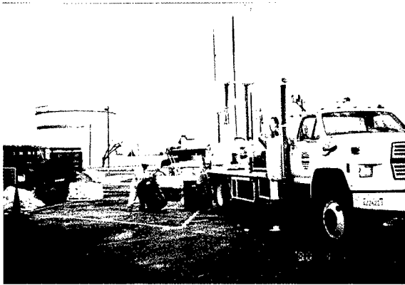
Photo 3. Mobilization of support equipment.
