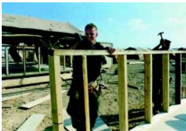
Our enhanced beddown capabilities include this Harvest Falcon equipment, part of a 1,100-person housekeeping set of tents, electrical generators, and billets.
