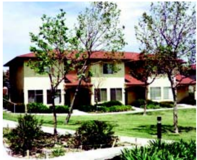
The renovation and construction of military housing units is key to our quality of life initiative to provide safe, affordable housing.
