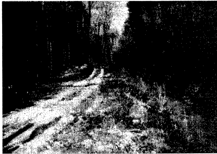
Figure 4-4. Single-bank construction. The visual effect would have been improved if clumps of trees had been left at intervals along the modified bank
