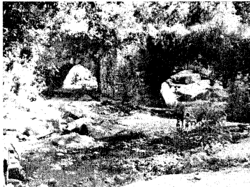
b. Espada Aqueduct in 1977
