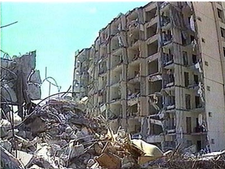
Damaged Barracks in Saudi Arabia
