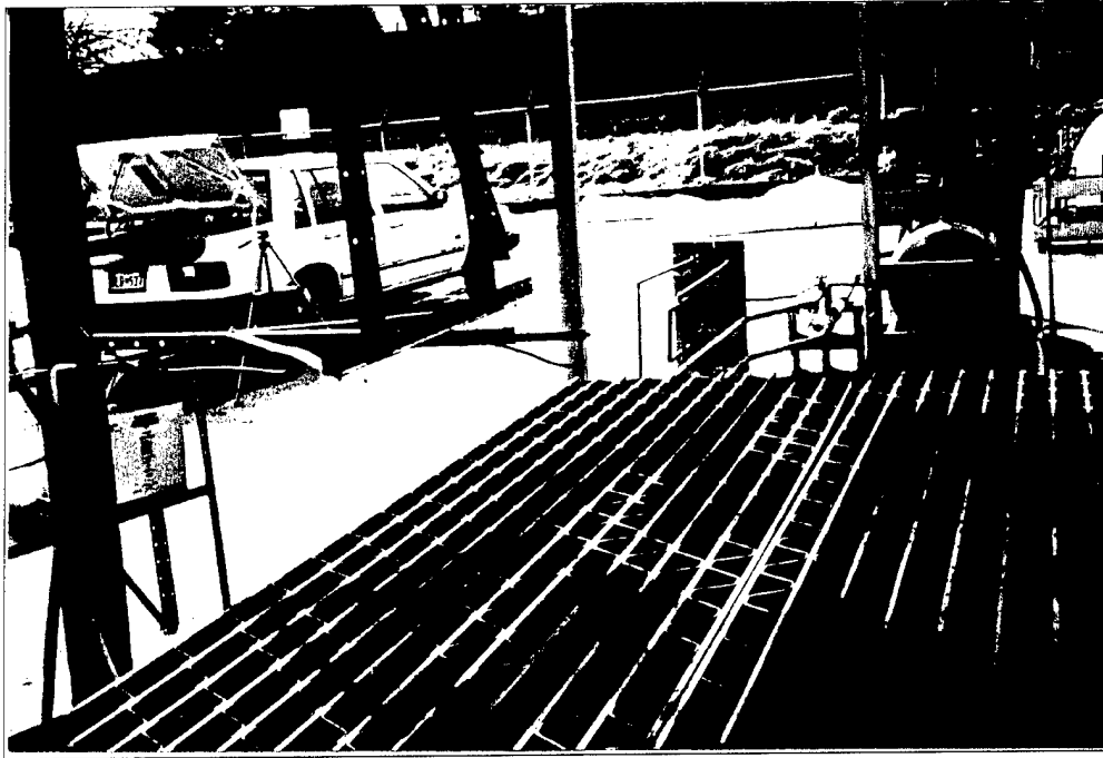
Figure 4-19. Grating assembled over burner.
