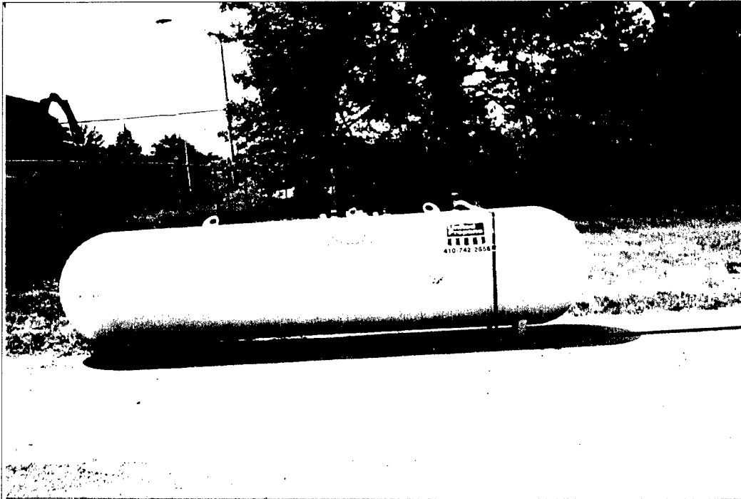
Figure 2-3. 1,000-gallon propane tank.
