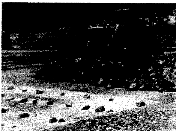
Figure 10-3. Placing a lift in the Cerrillos Dam test fill (Note the marking of the previous lift surface with plastic strips and lime)
