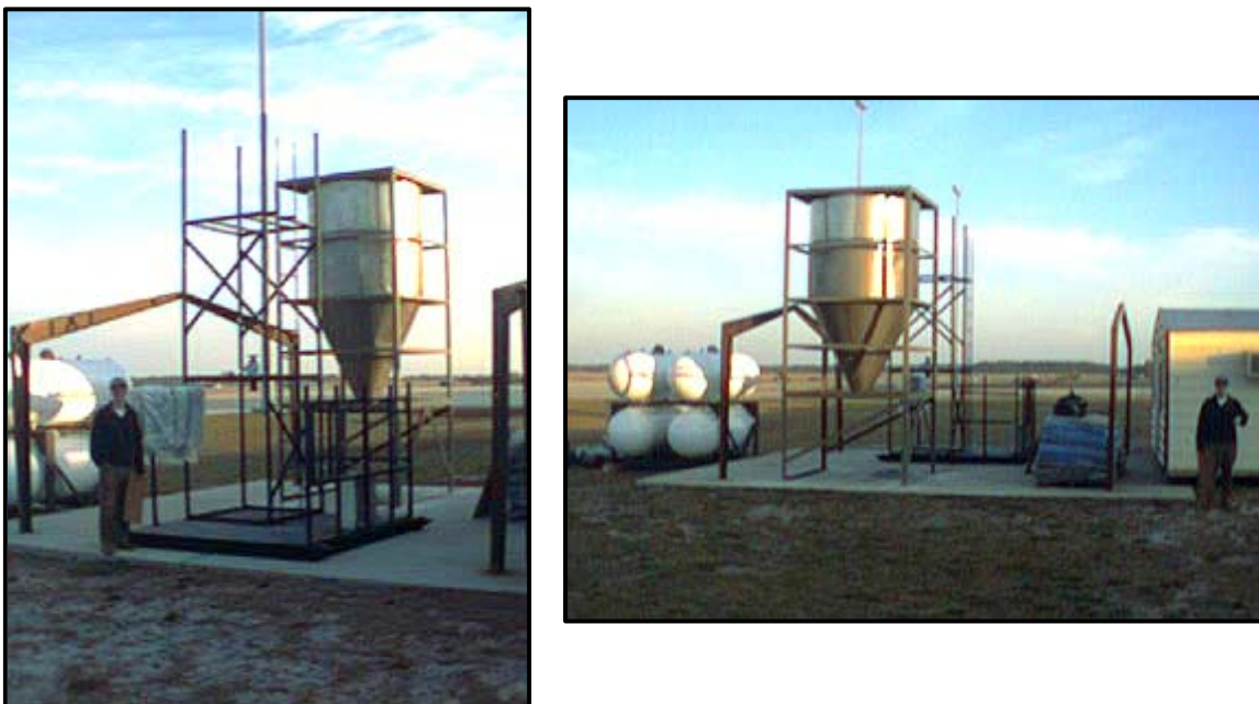
Figure 5. The adsorber vessel before the addition of the sidewalls and hoppers.
