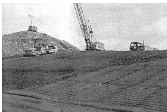
Figure 1-23. Reinforced RCC. Heavy welded wire mats can be placed in RCC to resist cracking and increase resistance to tensile stresses
