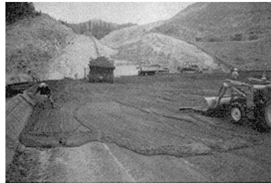
Figure 1-8. Application of mortar bedding
