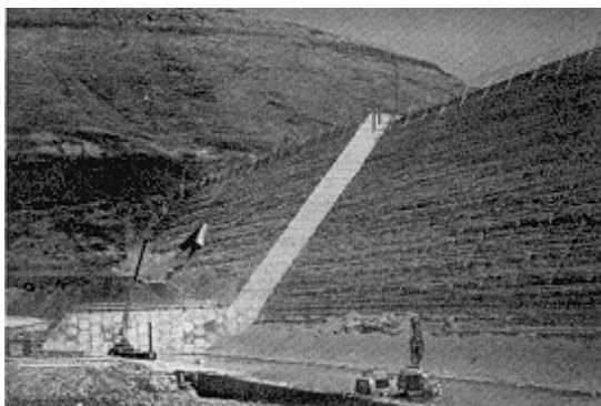
Figure 1-15. Unformed (D/S) surface finish
