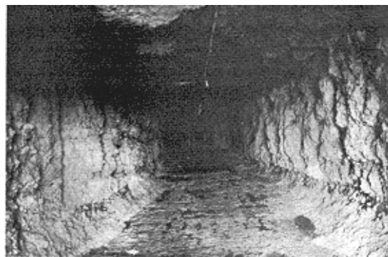
Figure 1-19. After excavation of the gravel/sand fill, protruding or loose RCC is removed. However, gallery walls are irregular and rough
