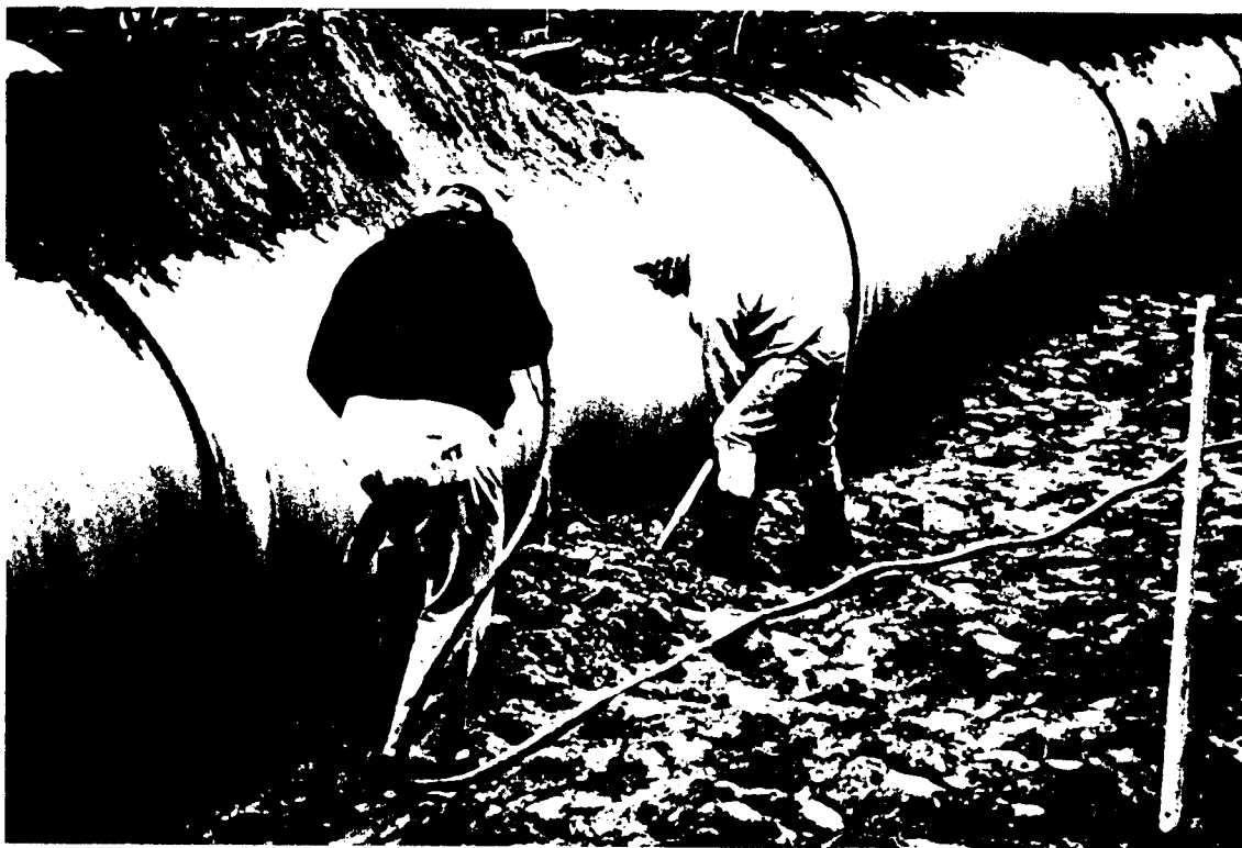
Figure B-1. Installation of FRP pipe
