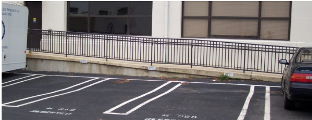
(a) Photograph of ramp.
