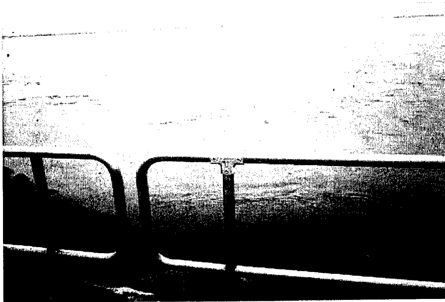
Figure 8-18. Bolted tee connection retrofit of fractured hand rail
