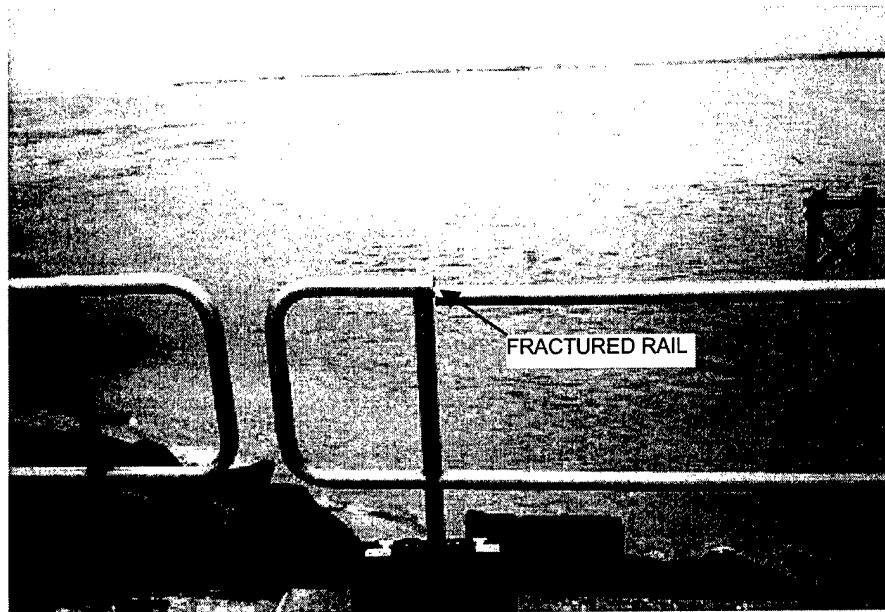
Figure 8-16. Cracked steel handrail
