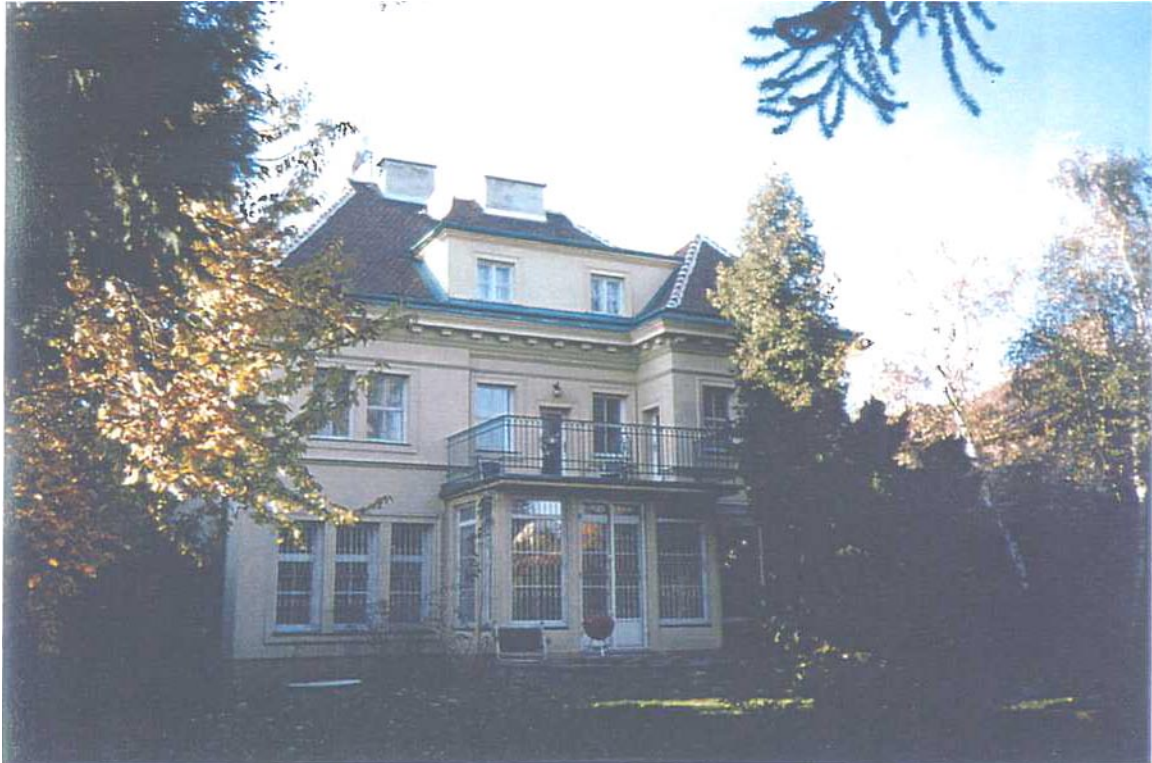
Figure 2: Vienna Residence (rear view)
