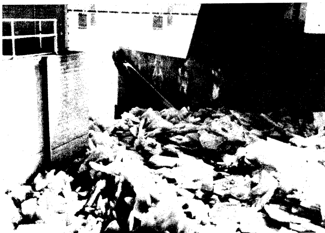
Figure 5-23. Ice on control gate
