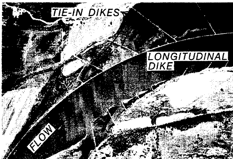
Figure 7-6. Longitudinal dike on Arkansas River
