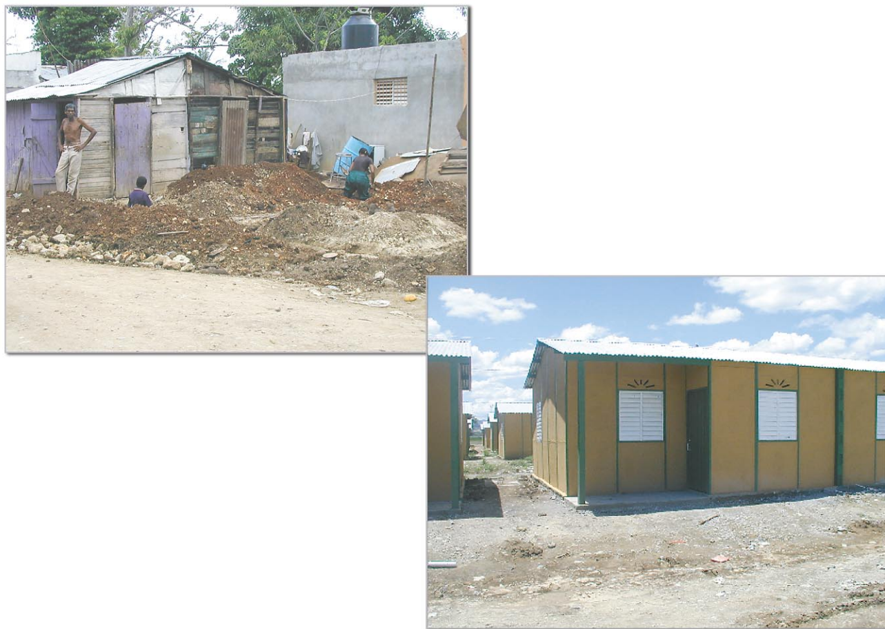
Figure 2: Damaged and Permanent Housing in the Dominican Republic
