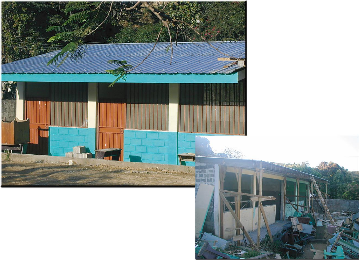
Figure 4: School Under Repair in Honduras
