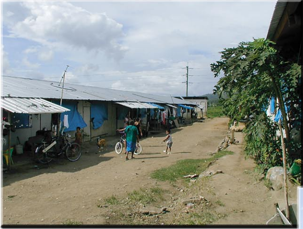
Figure 5: Temporary Shelters and Permanent Housing at El Pataste, Honduras
