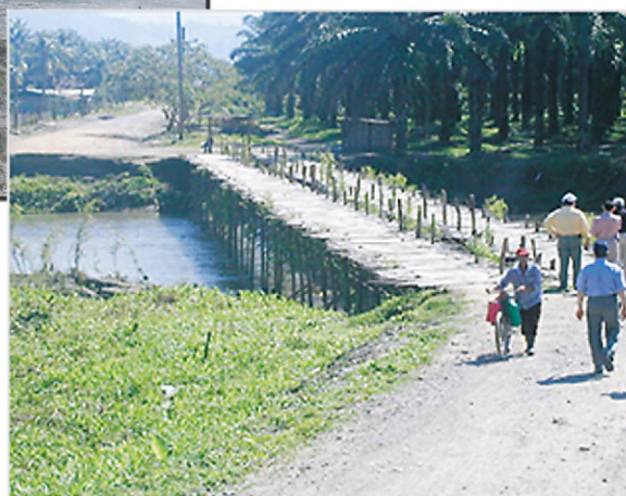
Temporary bridge erected after hurricane
