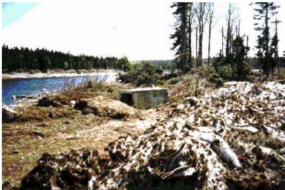
Figure 1. Gage house for USGS Gage No. 01010000, St. John River at Ninemile Bridge, Maine, following April 1991 ice jam. Note remaining ice debris, right.
