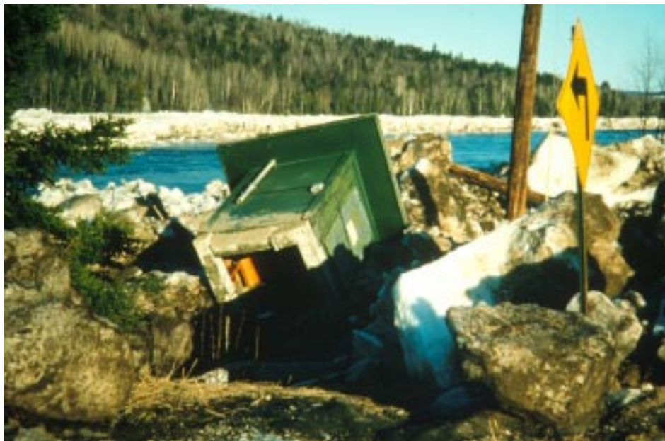
Figure 1. USGS gage house destroyed by ice at Dickey, Maine.
